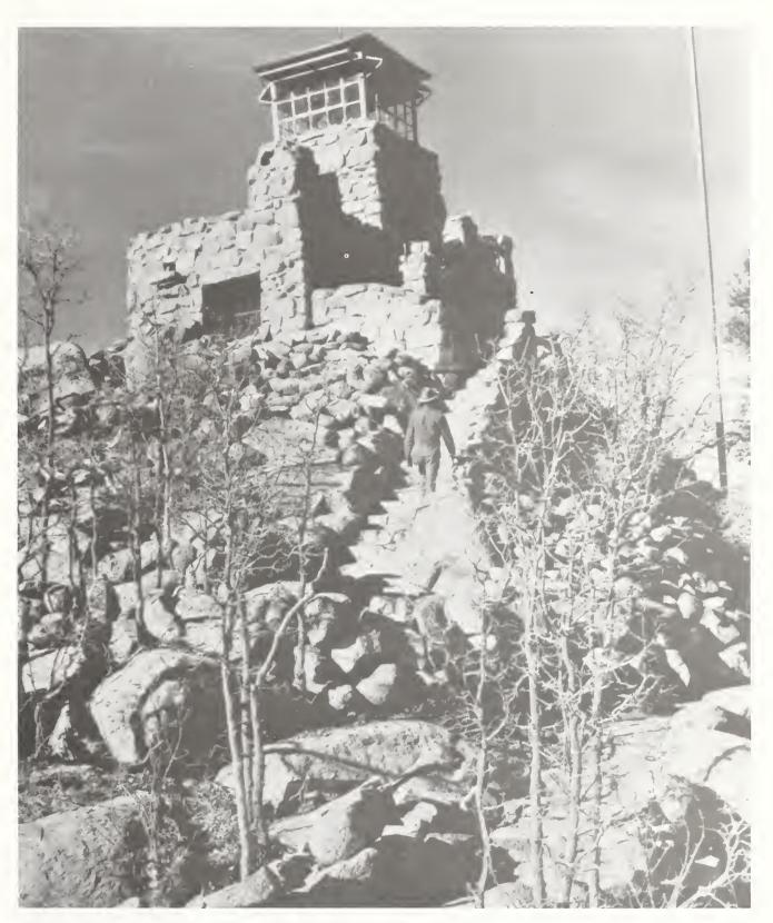
Figure 50. Monjeau lookout, constructed in 1940 on the Lincoln National Forest, New Mexico. This is perhaps the most unique lookout in the Southwestern Region. It combines a metal cab manufactured by International Derrick with a tower of native stone. It is the only example of a "rustic style" lookout in the Region. Photo by W. J. Mead made in 1941 (U. S. Forest Service 413954).
